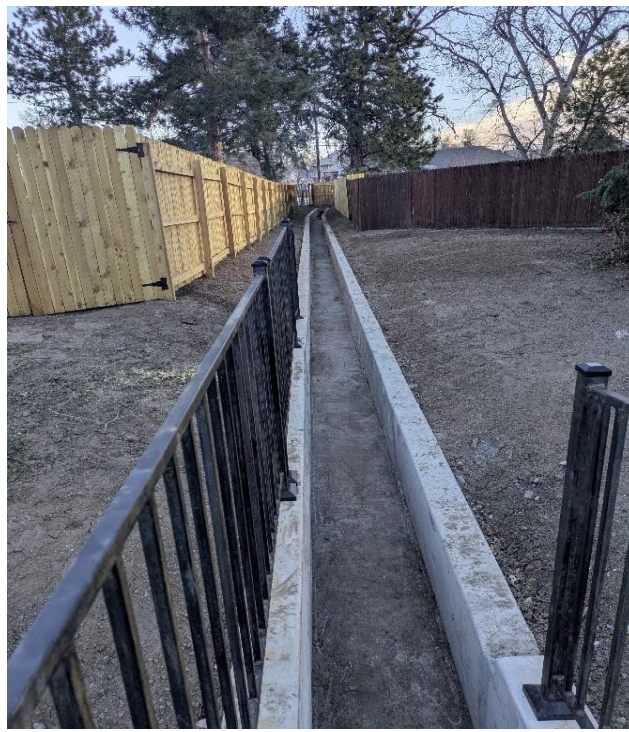
Concrete overflow channel within existing drainage easement
