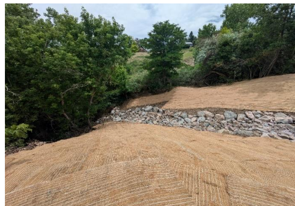
Riprap and erosion control blanket was installed to stabilize the slope
