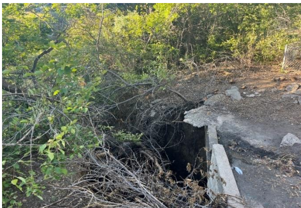
Shear drop off/Sink hole
