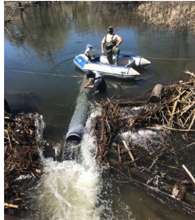
This interesting device, known as a “Beaver Deceiver,” is installed in the Bear Creek Greenbelt. It allows staff to better manage the beaver pond water level without triggering beavers to remove more trees to patch the dam.
