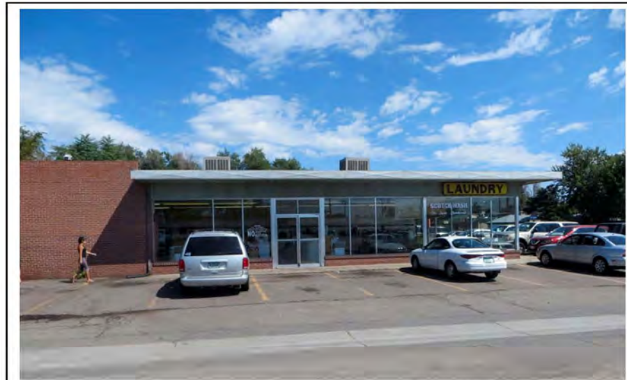
5JF.6527 – Looking North – Southern Facade. Scotch Wash Laundry. 1565 Carr Street. Photo ID: 5JF6527d. September 2014.
