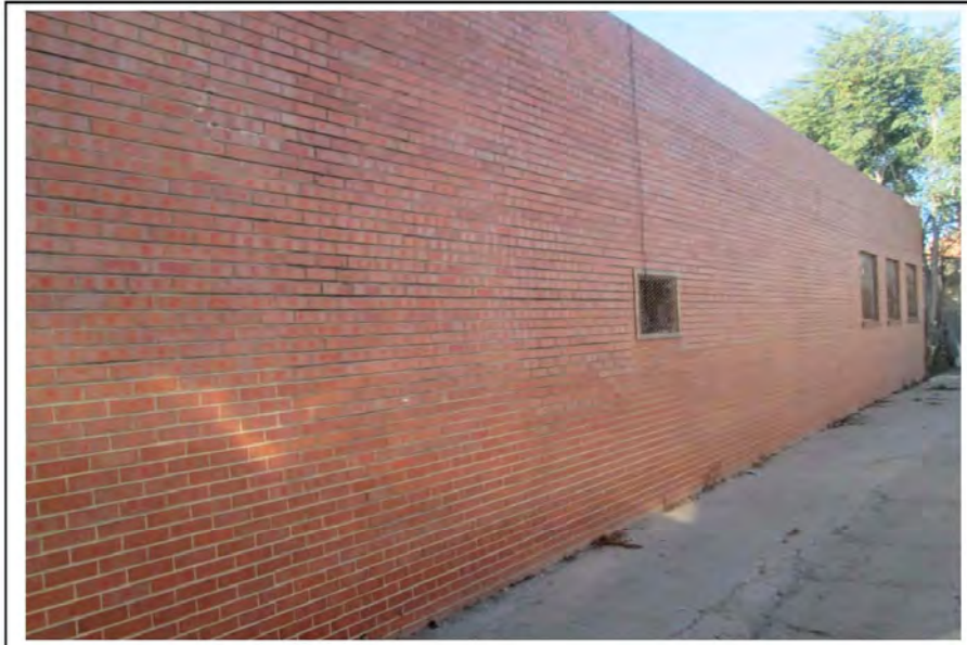
5JF.6527 – Northern facade. Looking Southwest. Scotch Wash Laundry. 1565 Carr Street. Photo ID: 5JF6527c. October 2015.
