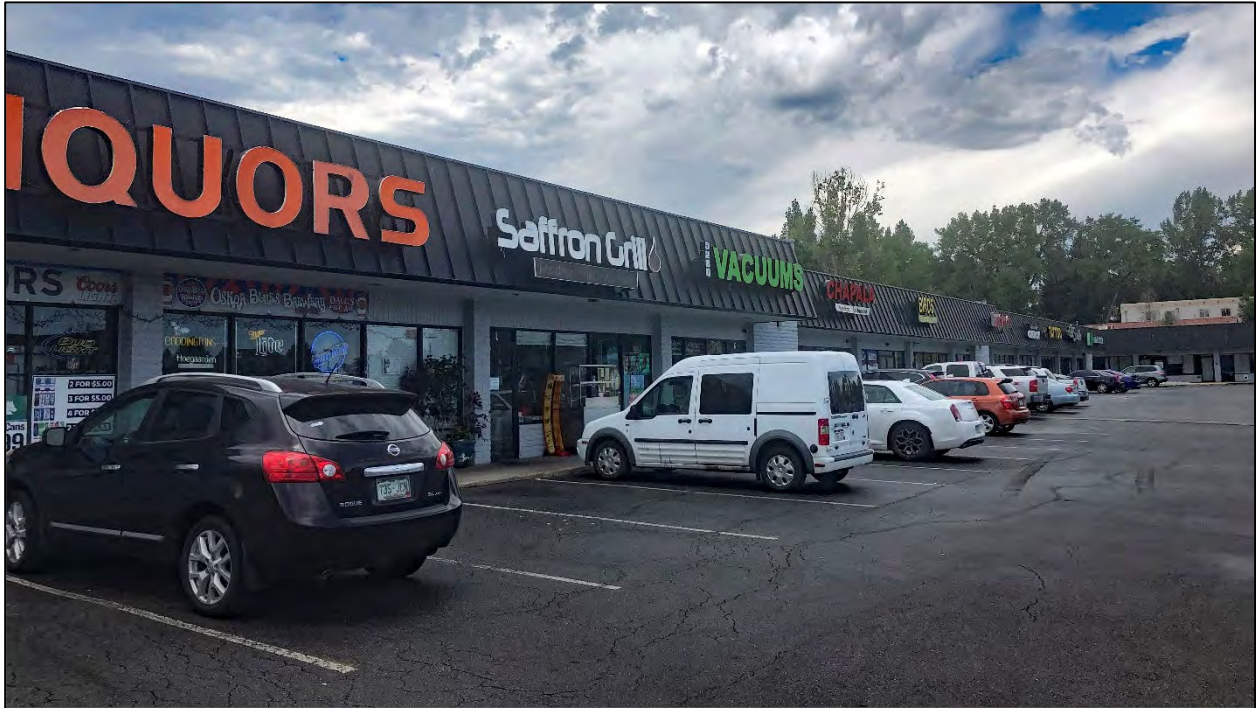
Figure 42. The L-shaped Parkridge Plaza Shopping Center opened in 1979. SOURCE: fieldwork photograph, August 2019, Front Range Research Associates, Inc., Denver, Colorado.
