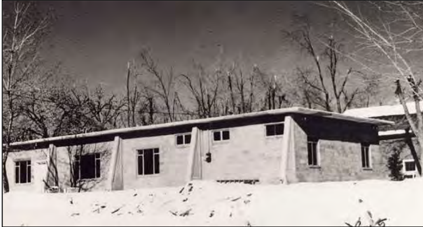
Figure 37. The Seventh Day Baptist Church purchased land at 2301 Wadsworth Boulevard and erected a concrete block fellowship hall with buttresses. A sanctuary to the east was added in 1969. St. Rafka's Maronite Catholic Church now owns the property. SOURCE: Pictorial History, Denver Seventh Day Baptist Church, website.
