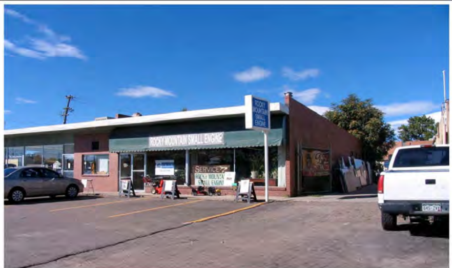
5JF.6527 – Looking southwest at eastern facade. Scotch Wash Laundry/Rocky Mountain Small Engine. 1565 (1575) Carr Street. Photo ID: 5JF6527b. September 2014.
