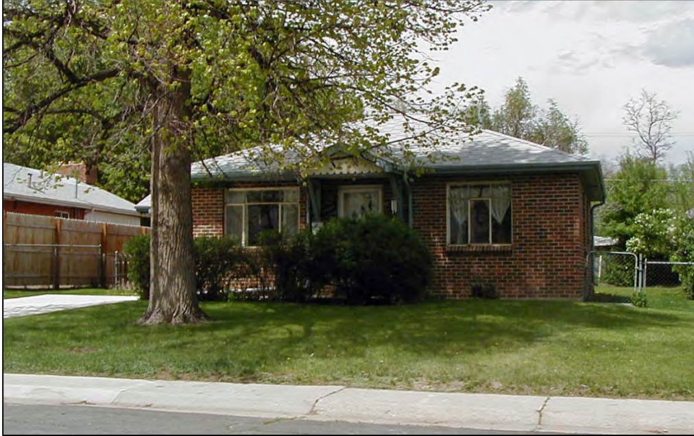
Figure 31. The 1949 Summers Resubdivision includes both sides of West 17 th Avenue between Yarrow and Allison Streets and contains several examples of small, one-story, brick dwellings, such as 7821 West 17 th Avenue built in 1949. SOURCE: Jefferson County Assessor photograph.
