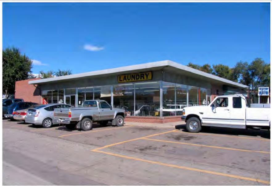
5JF.6527 – Looking Northwest at southern facade. Scotch Wash Laundry. 1565 Carr Street. Photo ID: 5JF6527a. September 2014.
