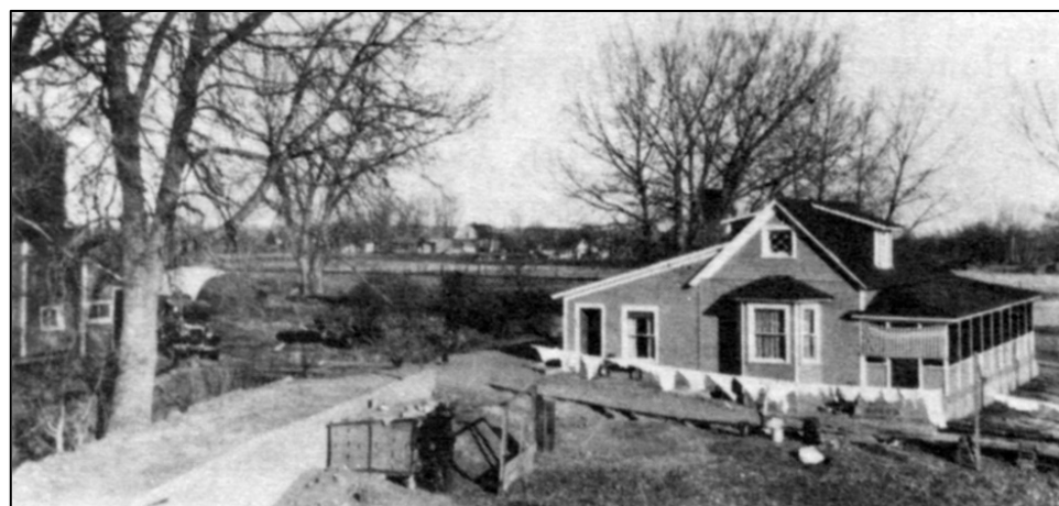
Figure 28. Laundry is drying in this view of the ca. 1913 frame farmhouse at 8300 West 18 th Avenue (extant but altered). It became the home of Arthur B. Johns in the 1930s. SOURCE: Wilcox, 76 Centennial Stories , 109.
