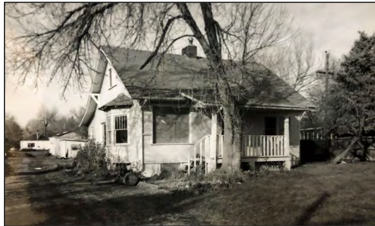
Figure 22. The 1928 house at 2501 Allison Street was part of an agricultural enterprise that raised pigs and chickens. SOURCE: photograph collection, Margaret L. DeLuca, Lakewood, Colorado.
