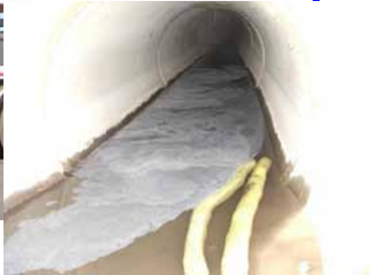
Washing out a concrete truck into the storm sewer and the results in the pipe.
