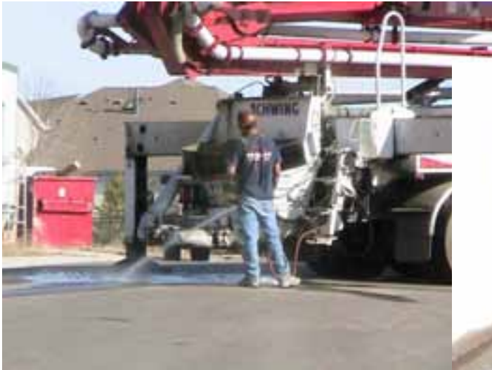
Washing out a concrete truck into the storm sewer and the results in the pipe.
